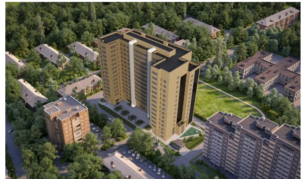
Fig. 3. Integration of the safety capsule into the architectural and planning structure of a 16-story residential building
