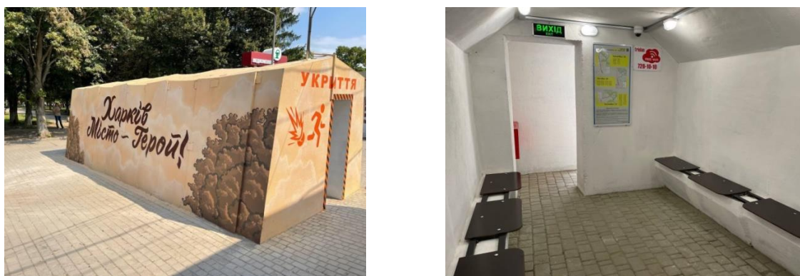
Fig. 2. Prefabricated protective structures at public transport stops in Kharkiv
